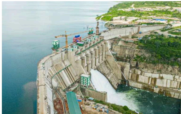
Julius Nyerere Hydropower Station at Rufiji
